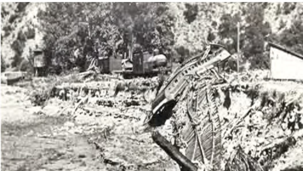
Above — Fallbrook station after January 1916 flood. Rails twisted and useless for miles. Trains never ran again in canyon. (Fallbrook Historical Society Photo used with permission.)
