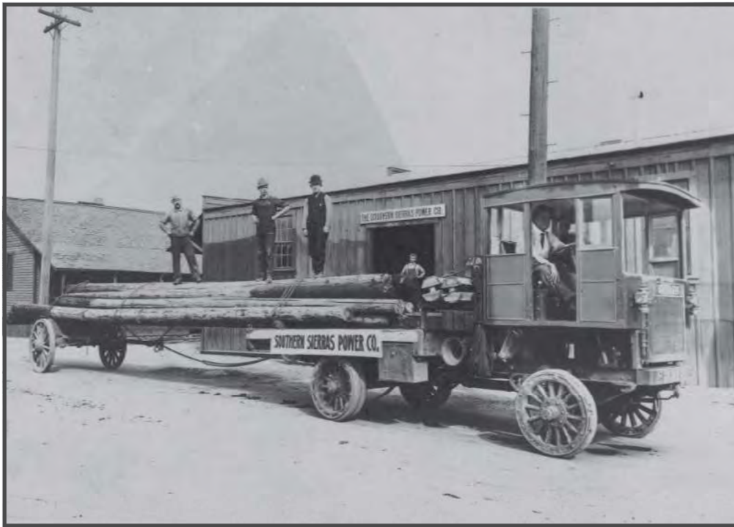
In 1913, poles were delivered to Elsinore for the construction of the transmission lines. Source: The Huntington Library Digital Archives
