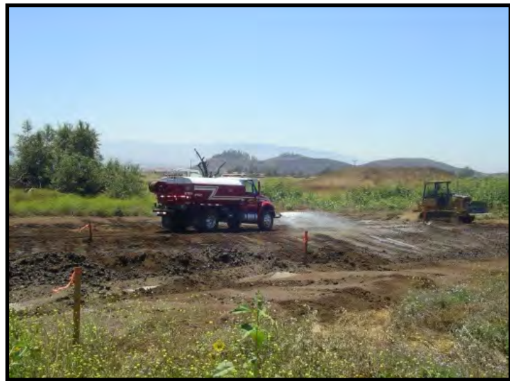
Department personnel graded pad for temporary Station #4.
