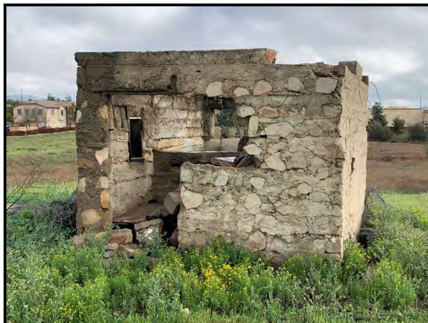
The Rail Pump House, Photo by author (March 11, 2020)
