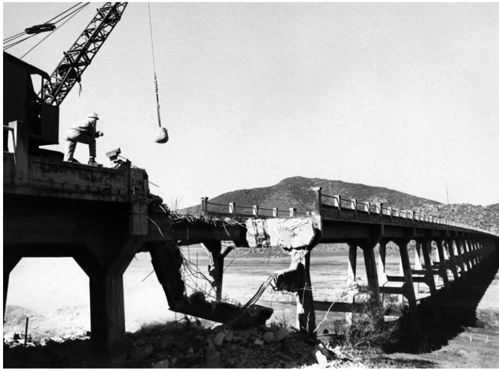
1968 Demolition of Bernardo Station Bridge Cost: Estimated $21,000
